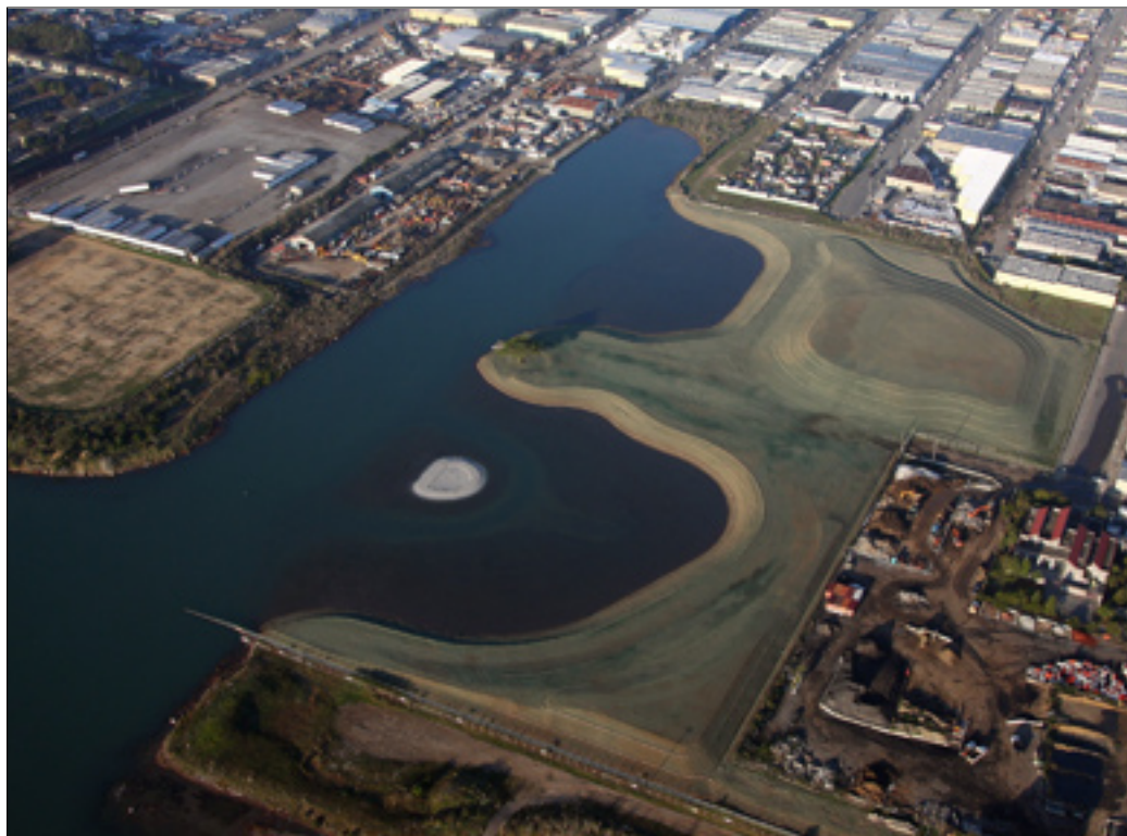
An aerial view of the Yosemite Slough Wetlands Restoration Project from December 2011 shows newly-laid hydro-seed. The aqua green seeds have now turned a golden yellow in the sun. Photo courtesy Top Grade Construction, Inc. 2011.
